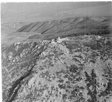
Aerial view of relay station at Kuri
