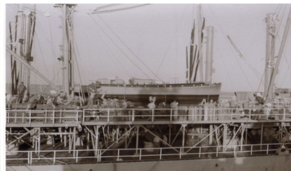
Guadalupe's maze of Pipes & Valves
